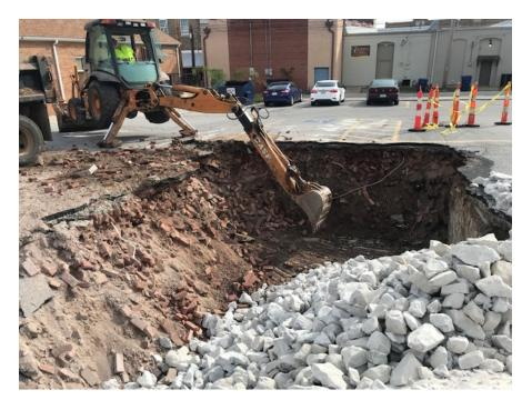
Waste Water and Public Works crews have been working to make some long needed repairs to the **Robin Ridge lift station** off of North Red Bird. We have fought water drainage issues there for years. The access was changed last year to keep city crews from having to go through a private drive and gate to get to it. Now we have concreted in the drive and preparing to pave the entrance that will channel the water and stop the erosion.
